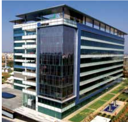
NetApp, Bengaluru - innovative office spaces
